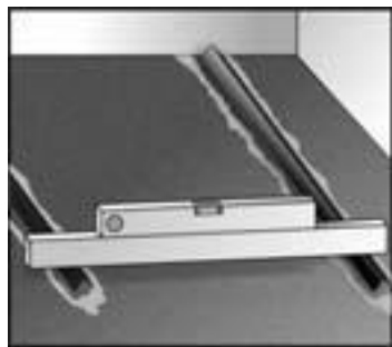
Figure 8 Making guiding rails
