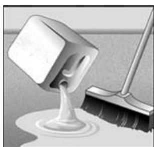
Figure 18 Applying the primer layer
