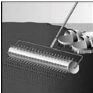
Figure 22 Mortar mix distribution with a spiked roller
